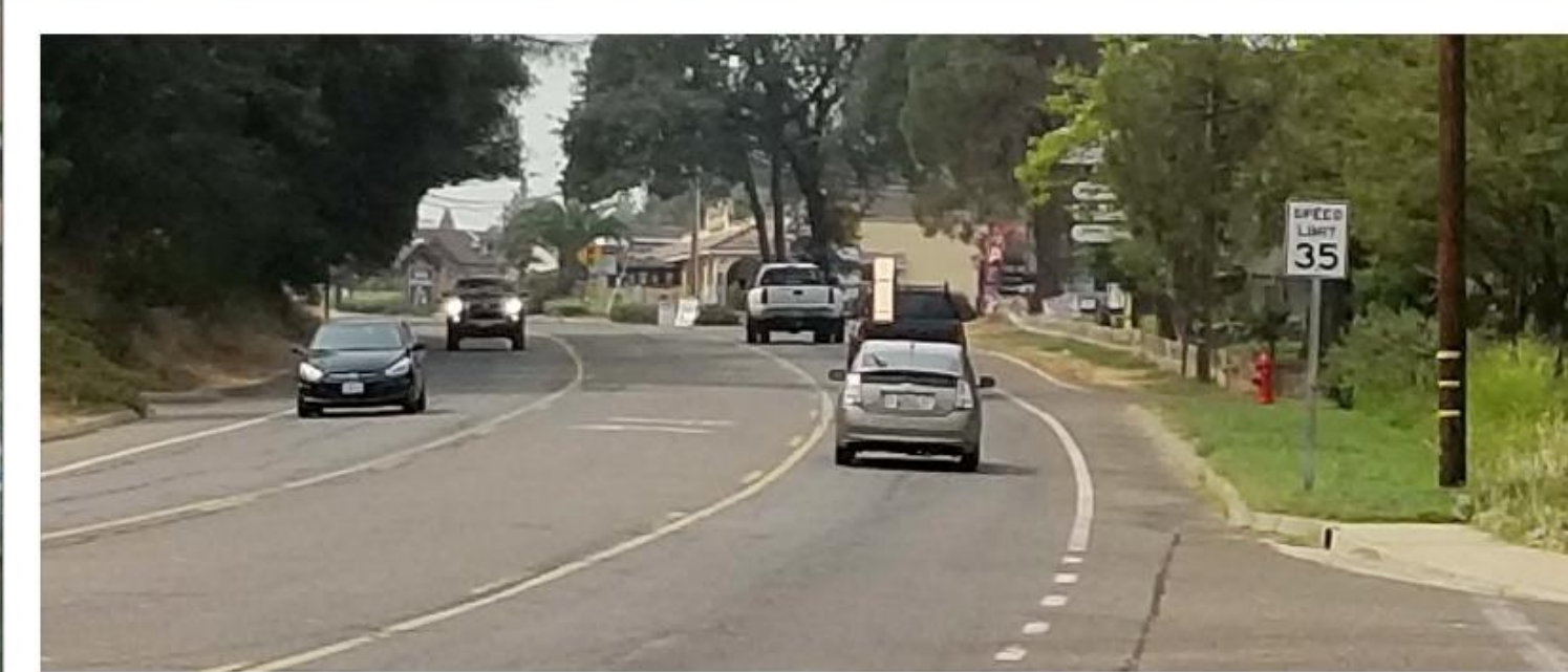
Barrier #3: Substandard bike lanes - 10,200 feet total
