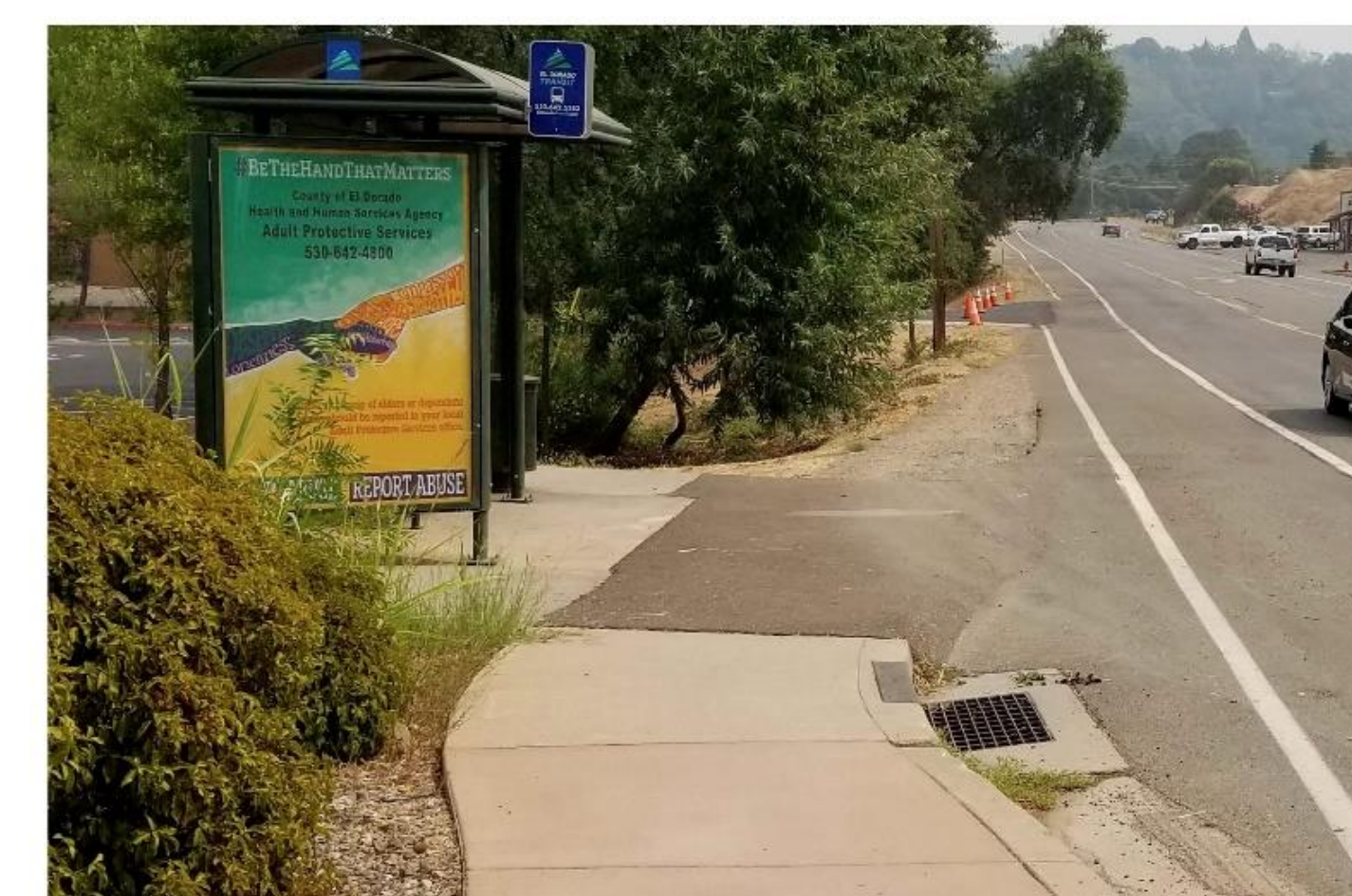
Barrier #5: Substandard (non ADA compliant) curb/sidewalk ramps - 12 total Barrier #6: Substandard Transit Stop - 3 total
